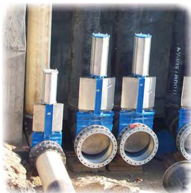
Mixing chamber installation
