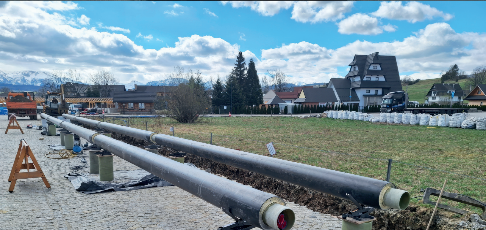
Geothermal pipeline, DN150, PN16, 2024
