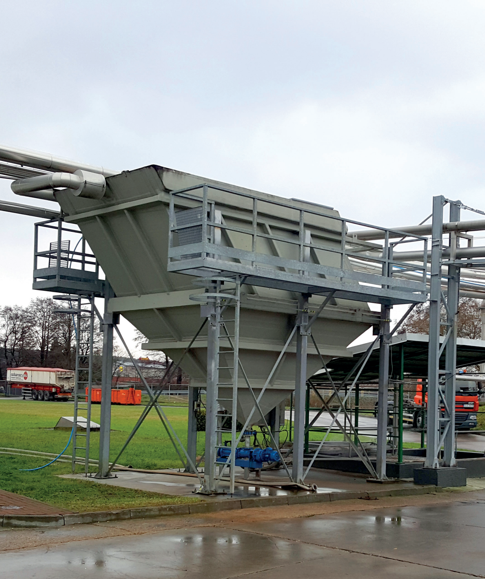
Lamella apparatus 12m 3 /h, food industry, 2016
